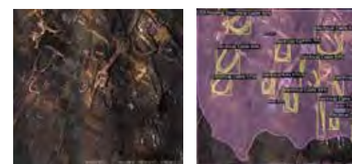
Figure 3: Detection of CRD Housing Support and Electrical Cables in Fukushima Daiichi: a) original raw image and b) prediction results after analysis with trained deep learning model.
